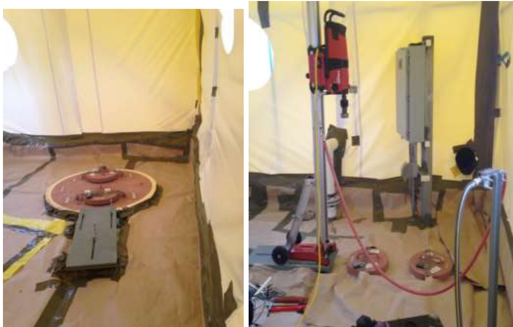
Fig. 6. Slotted mounting plate at an SDU 2A camera port (left) with drill rig installed (right).
