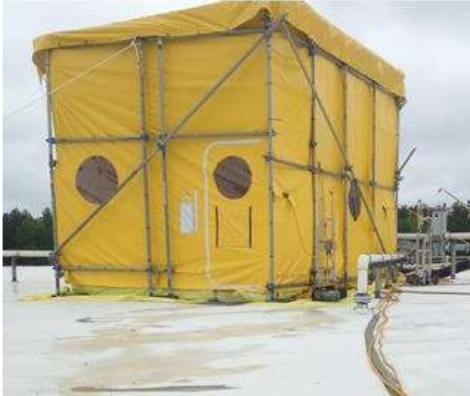
Fig. 5. Contamination Control Hut on SDU cell 2A.
